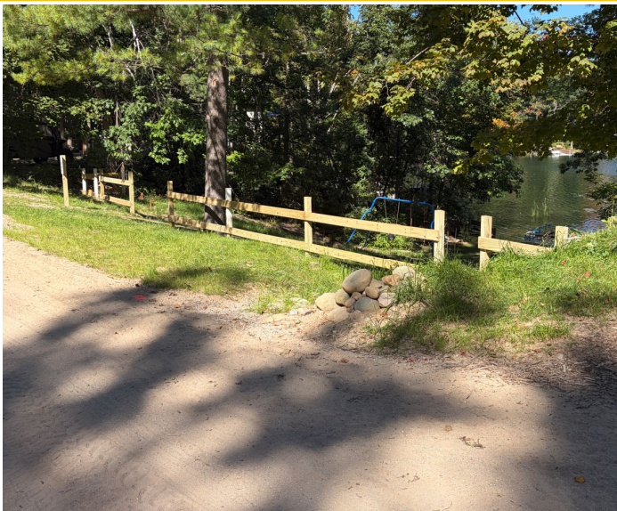
Work continues on repairing and painting park fences
